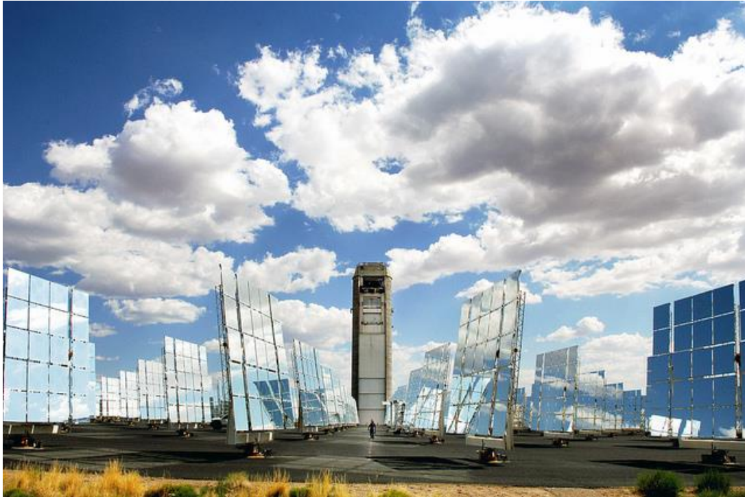
National Solar Thermal Test Facility (NSTTF)
